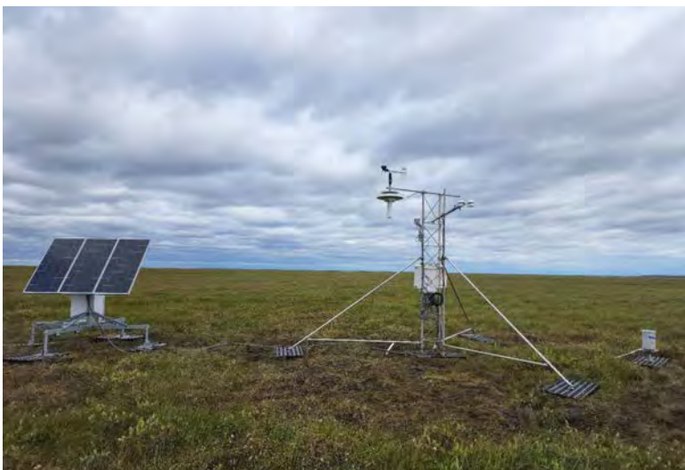
One of the FOCAL towers after installation.
